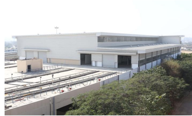
Rapid Metro Project (IL&FS), Gurugram
