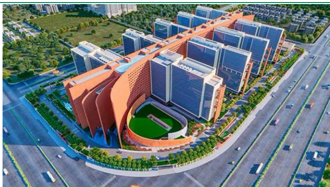
Fig 7: SDB - Comprises of 9 towers, with Ground + 15 floors
