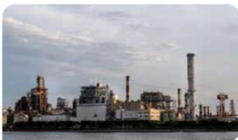
Primary &amp; Secondary structures for boilers &amp; turbine generators
