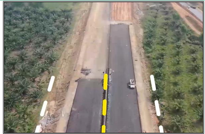
Fig 36: Various course of an under-construction road at AP-1 site*
