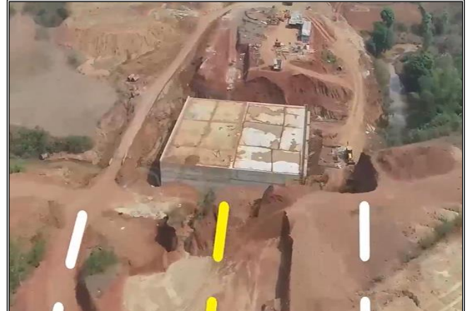
Fig 38: Showcases a minor bridge and equipment at OD-6 site*
