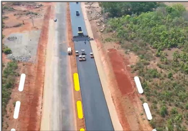
Fig 37: Surface course being laid with a pavement machine*
