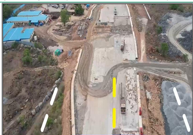
Fig 32: Package -1 site photos show box culvert and toll plaza*
