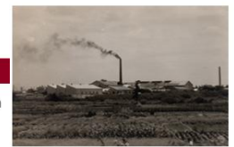
High-pressure laminate (HPL) plant completed in 1959
